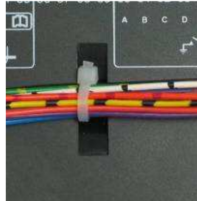
With Cable And Tie In Place
